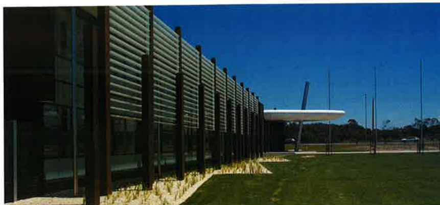
Located in Torquay, the Surf Coast Shire Council office presents a hallmark in environmentally sustainable design.
